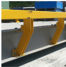
Side rails and steel ramps
